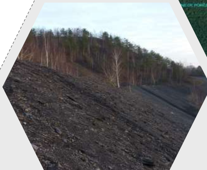
Wendel (57) – 17 000 kWc Mine de charbon
